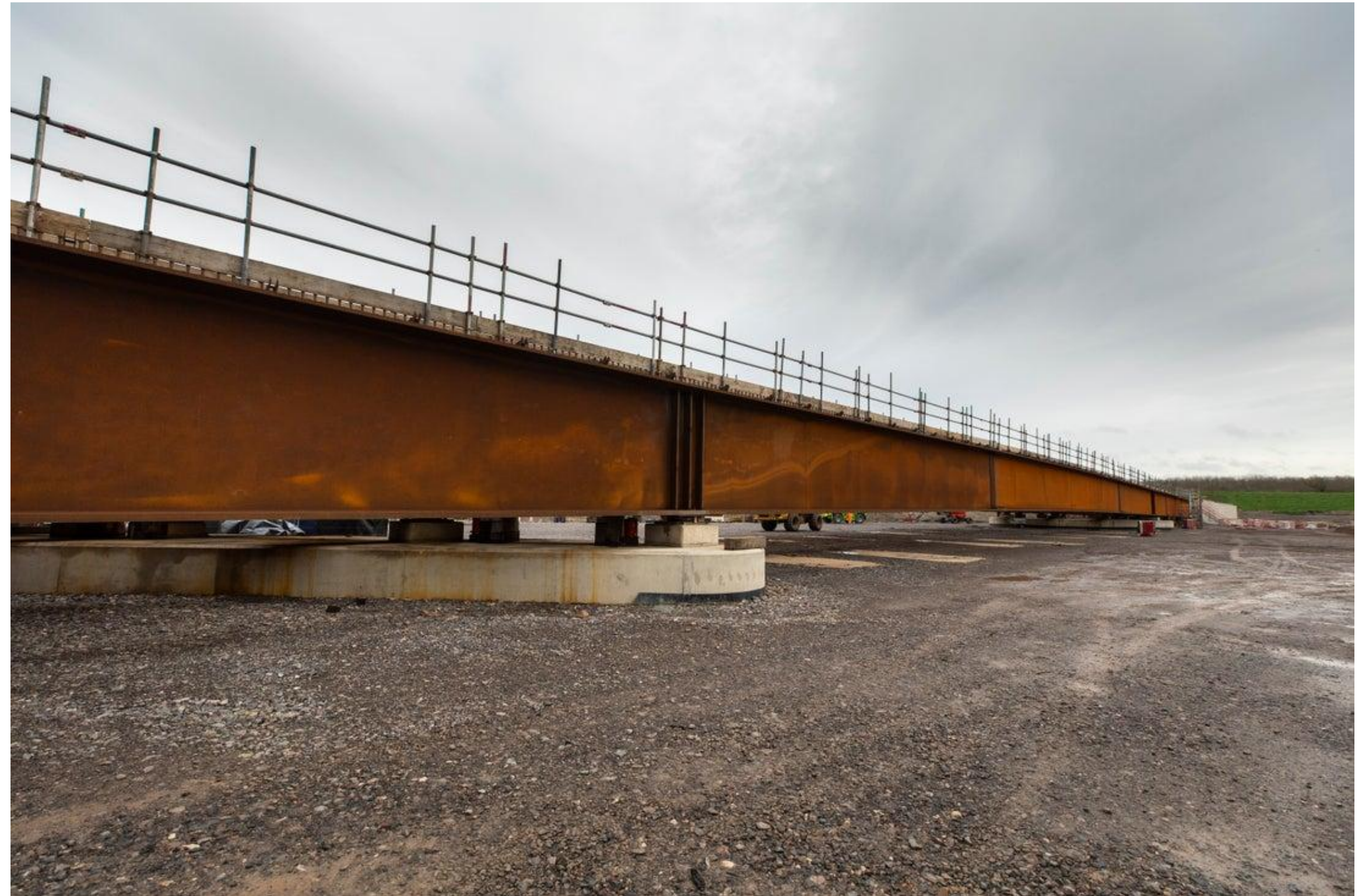
Nash Lee overbridge being lowered onto permanent bearings, November 2025
