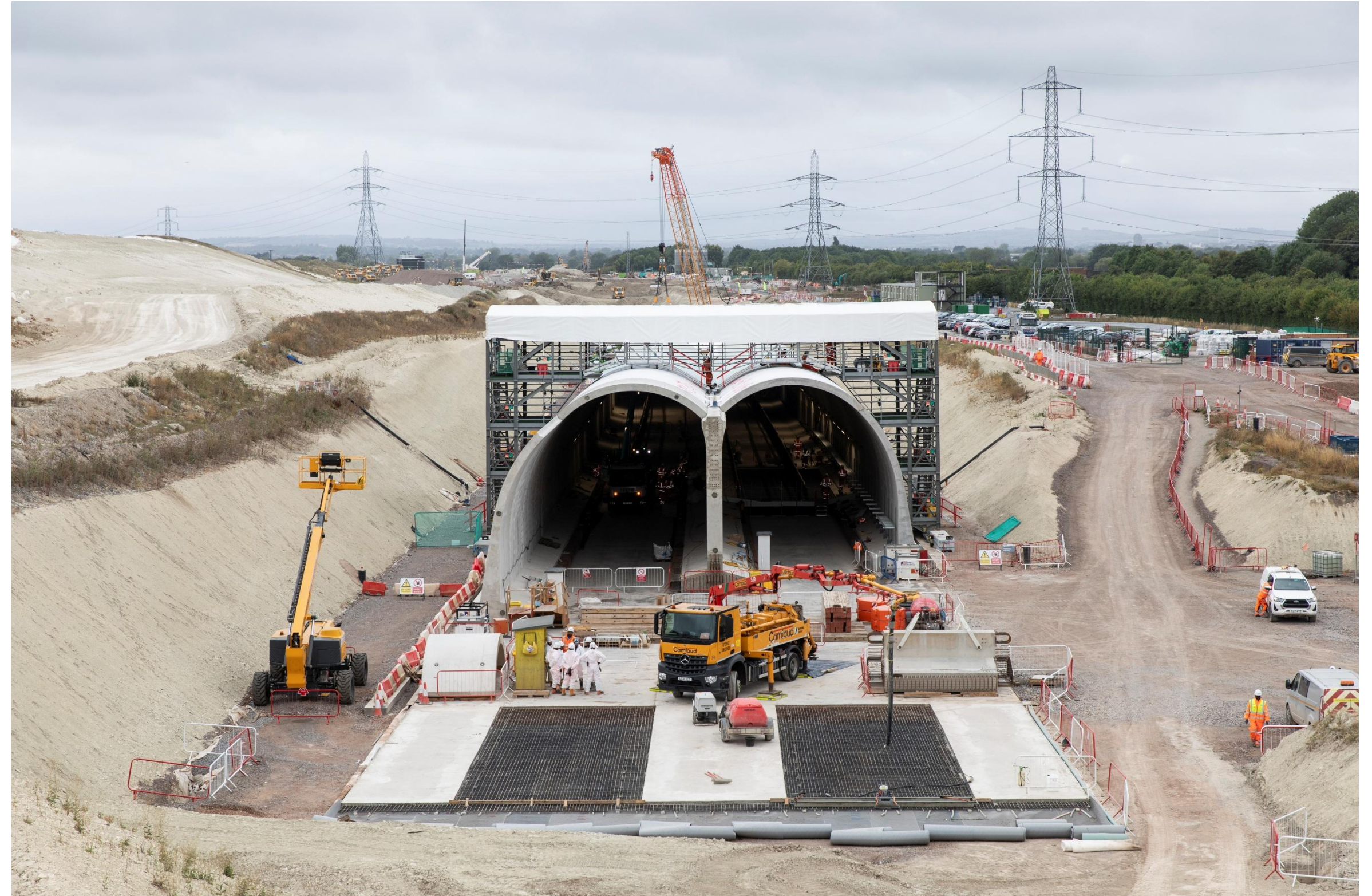
Wendover green tunnel from Ellesborough Road, Autumn 2025
