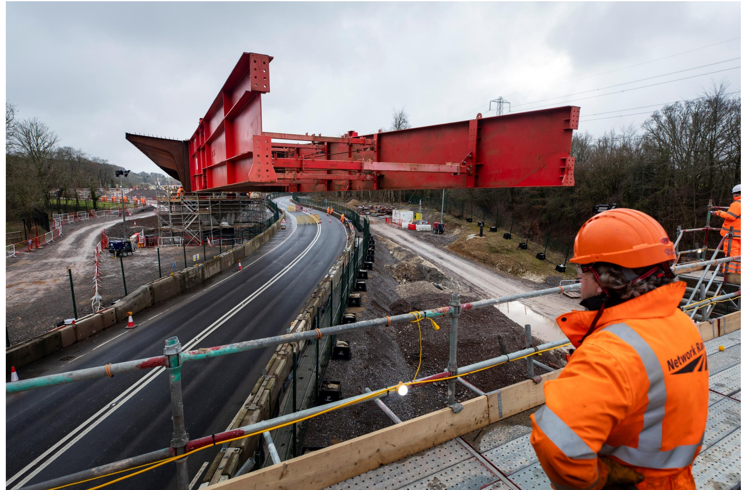
Small Dean viaduct during the deck slide in January 2025
