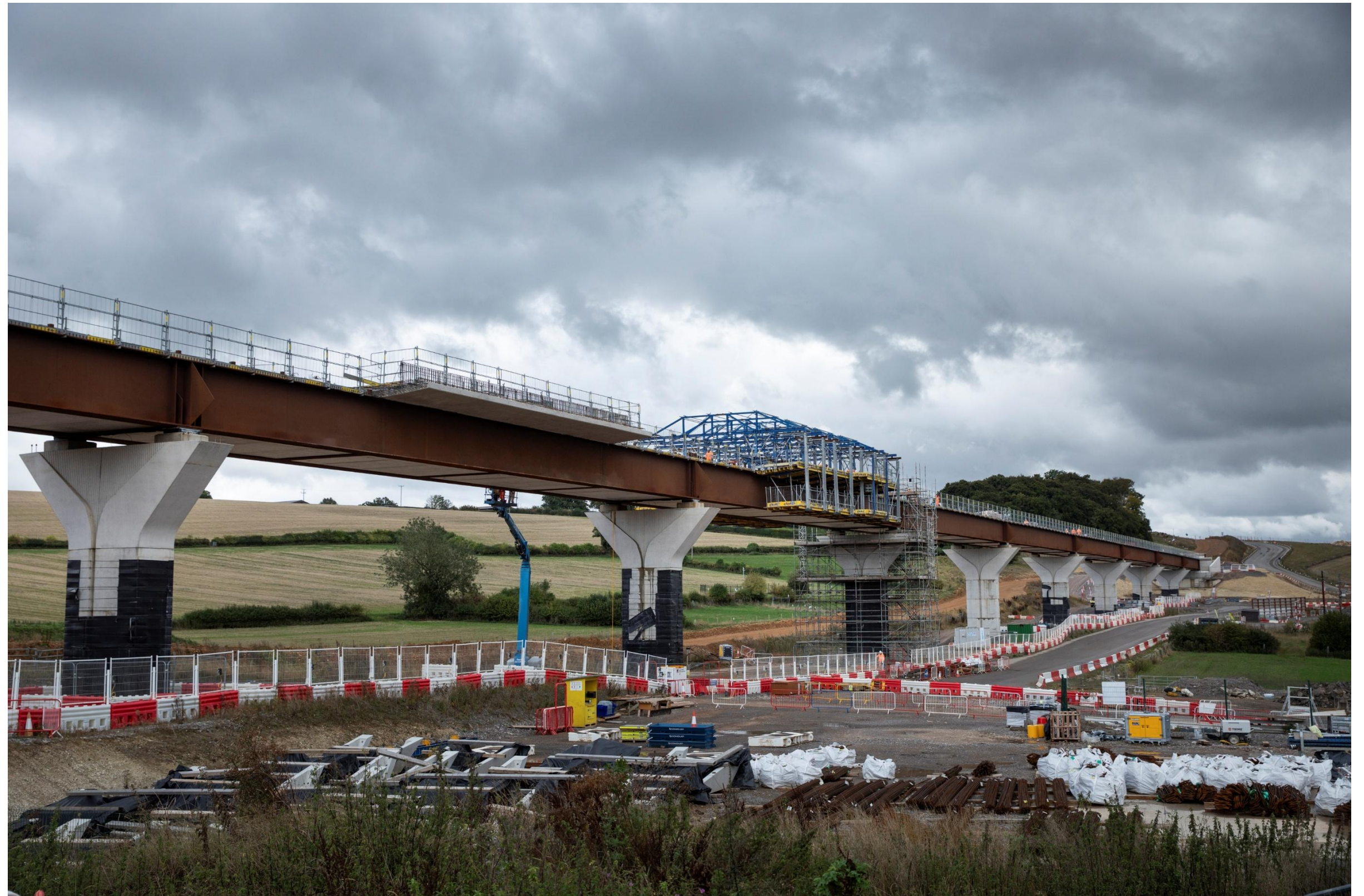
Wendover Dean viaduct, Autumn 2025
